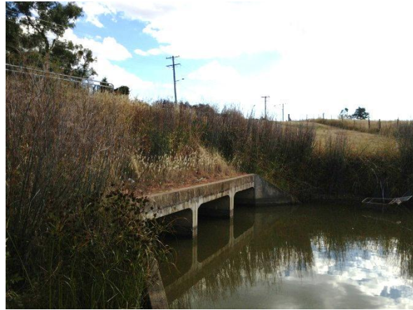
PICTURE 5 – BARNES GULLY - CULVERT UNDER SCOTT ROAD
