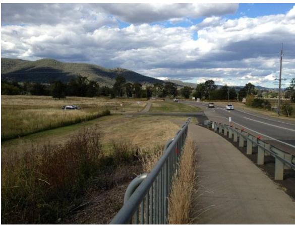
PICTURE 6 – LOOKING EAST ALONG SCOTT ROAD FROM BRIDGE ACROSS BARNES GULLY
