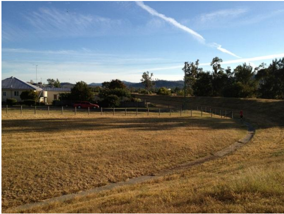
PICTURE 10 – DWELLINGS TO THE NORTH OF THE SITE PROTECTED BY AN EXISTING LEVEE BANK
